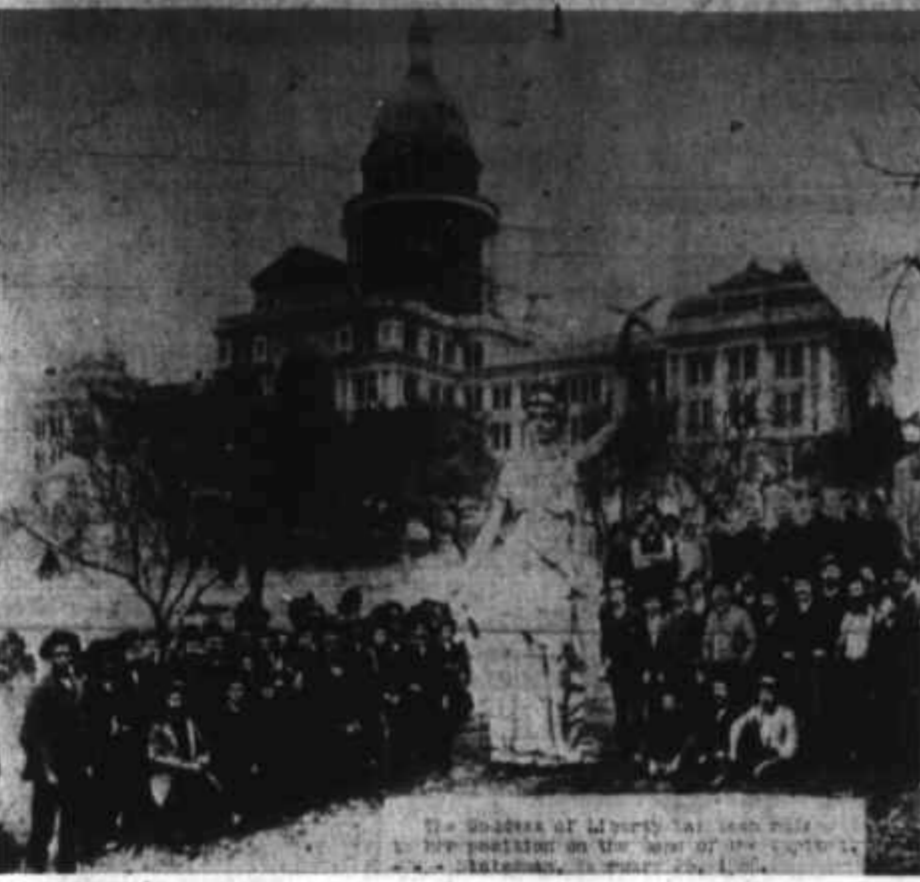
Workers are shown at the time the Goddess of Liberty was raised at the top of the State Capitol building over a century ago. Austin State photo.
